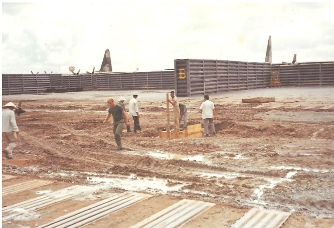
Doug Emch & Fred Benda & Crew working on PVC Matting and drainage for the 8th Airport taxi way.
