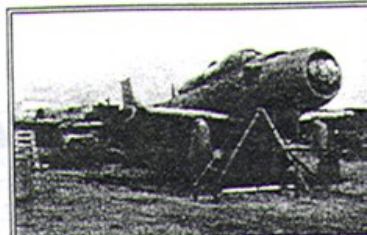
AFLC kept a detachment at ISN to repair aircraft which were damaged beyond my capability to repair. They were real "wizards" at bringing life back into combat damaged aircraft such as this A1E "Skyraider." These were former Navy attack bombers. The Navy called them AD. A for attack and D for Douglas. They had huge R-3350 Curtiss-Wright 3000 hp radial engines. (Photo from TBM)
