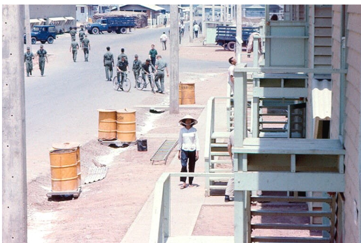
Looking North from the 1200 barracks area. The second building on the left, just past the jeep, is Dining Hall #4. The small shelter at right center, just beyond the parked truck is a shuttle bus stop.
