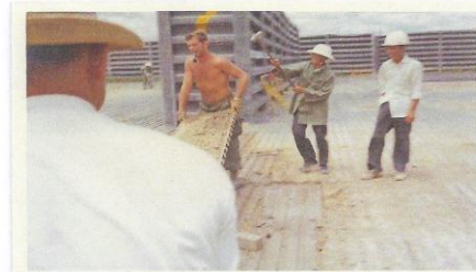
Fred, Doug Emch and crew installing matting and drainage for the 8 th Airport Taxiway
