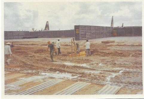
Fred, Doug Emch and crew installing matting and drainage for the 8 th Airport Taxiway
