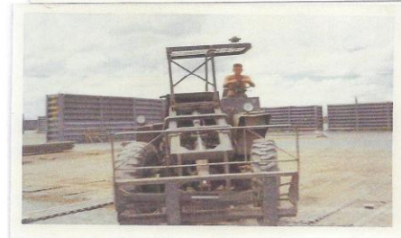
More picture working on the 8 th Airport Taxiway, 1200 area.
